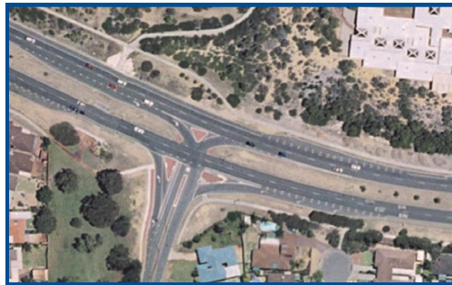
Figure 1 An Example of a Seagull Intersection in Western Australia (Radalj et al. 2006)
